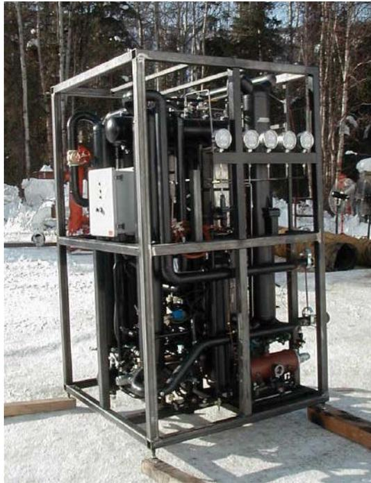
Figure 8: 16 ton Thermochiller installed at Aurora ice hotel (Courtesy: Don Erickson, Energy Concepts).
