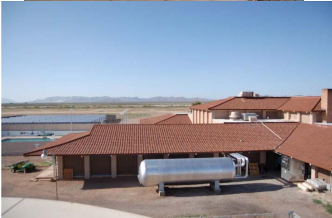
*Figure 10: 60 ton solar-fired Helichiller (above) with storage tank (below) (Courtesy: Don Erickson, Energy Concepts).*
