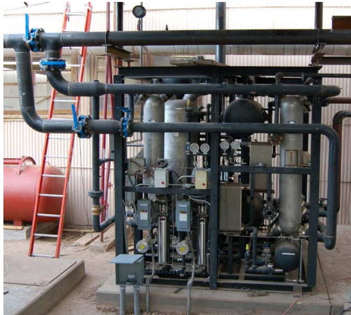
Figure 7: 160 ton Thermochiller (Courtesy: Don Erickson, Energy Concepts).
