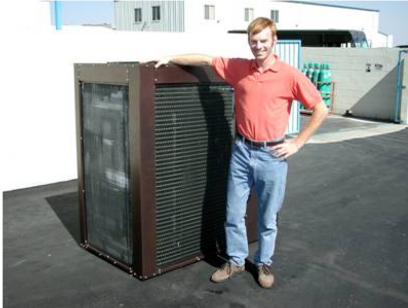
Figure 6: Ammonia-Water 5RT Gas Fired Air Conditioner (Courtesy: Uwe Rockenfeller, Rocky Research).
