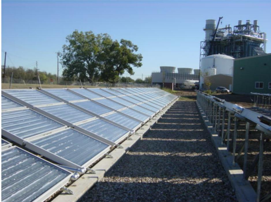
Figure 12: Austin Energy solar collector field for polygeneration (Courtesy: Solargenix).
